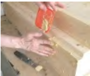
Applying Makeweight Dough (WOOD FILLER)
